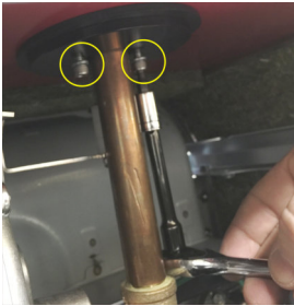
2e-1/2 Install supplied 2 clamp halves on top of unit then tighten 2 clamp bottom 5/32" socket head bolts on underside. USE CAUTION- BEWARE OF SHARP EDGES ON SHEET METAL FRAME
